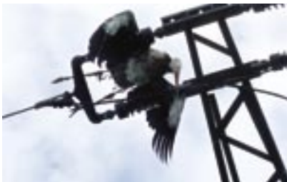
With its extremely long wings the White Stork has bridged the insulators and was killed by the electric flow through its body.
