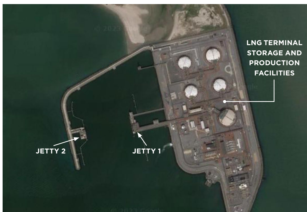
Figure 44. Map of the LNG Terminal with the marked locations of Jetty 1 where Case A was measured and Jetty 2 where Cases B and C were measured (Maps data: Google, ©2022, 2023 CNES / Airbus, Maxar Technologies).
