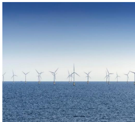
Abb.1: Offshore-Windenergie (© imageBROKER.com / Markus Keller)
